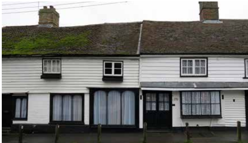
Figure 58: Grade II listed buildings with traditional white weatherboarding and clay roof tiles on Church Street.
