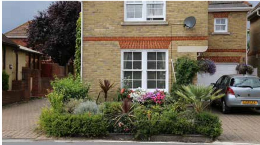
Figure 60: Yellow brick house with flat-arched red brick lintel, sash windows with white muntins, and slate roof.
