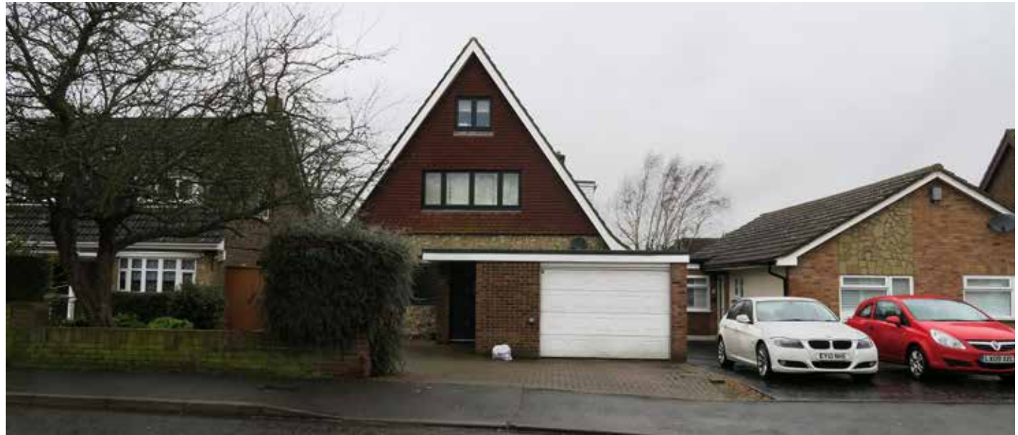
Figure 37: An example of variety in massing used for house frontages.
