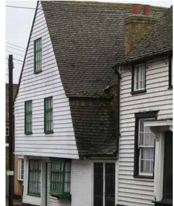
Figure 57: Longford House, a Grade II listed building with jettied upper storeys and painted window frames.
