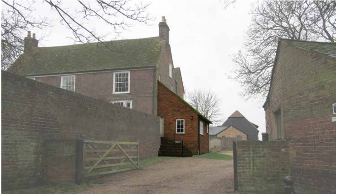
Figure 49: Successful side extension to a Grade II listed building.
